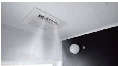
Hot water-type bathroom heater/dryer
