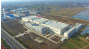
Shanghai Rinnai's new factory
