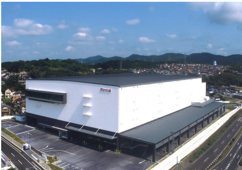
Kasugai Distribution Center (Kasugai City, Aichi Prefecture)
