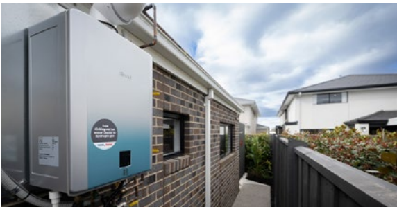
Testing of Rinnai's 100% hydrogen combustion water heater (Australia "Hydrogen House")
