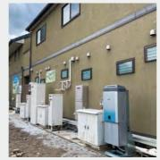
Installed 100% hydrogen-burning water heaters
