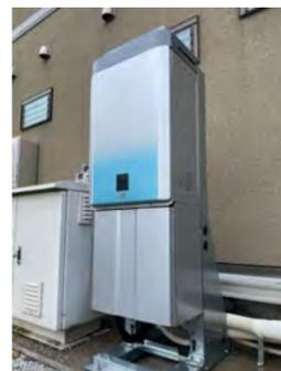
Testing of Rinnai's 100% hydrogen combustion water heater at Kitakyushu Hydrogen Town
