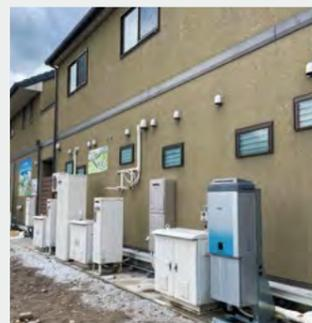
Installed 100% hydrogen-burning water heaters
