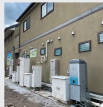
Installed 100% hydrogen-burning water heaters
