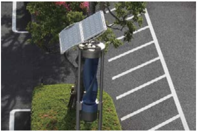
Compact wind and solar power generator (Head Office)
