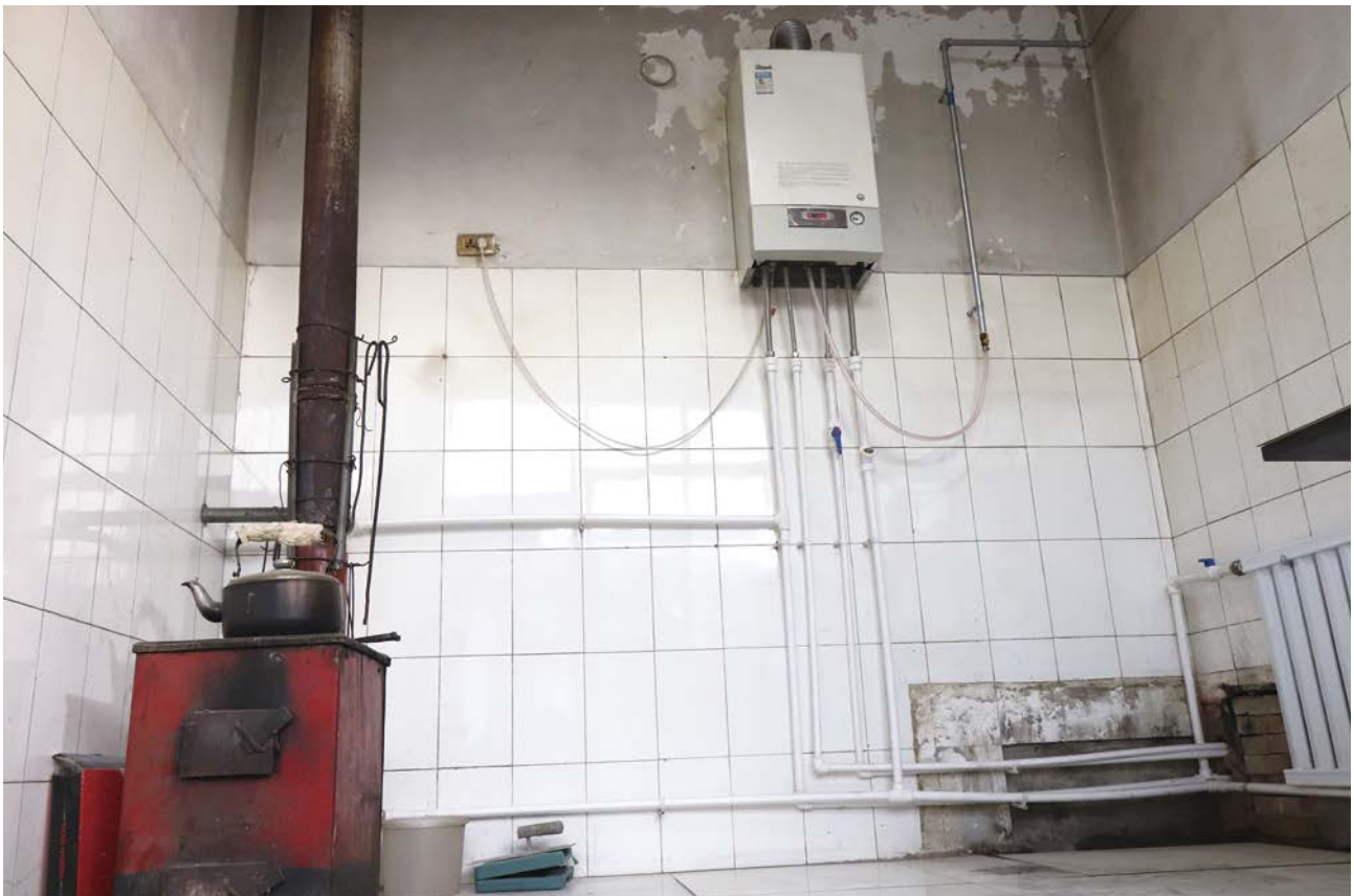
A gas boiler (top right) that replaced a coal-powered boiler used previously (bottom left)
