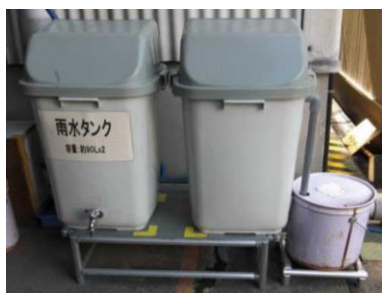
1) Rainwater tanks
