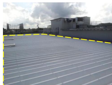
Area of the roof coated (corrugated panels on Factory 1)
