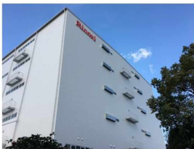
External view of East Japan Logistics Center
