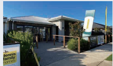
Hydrogen House (Victoria, Australia)
