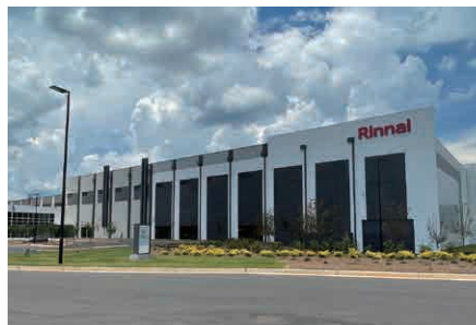
New plant of Rinnai America (Griffin, Georgia)
