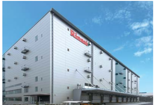
Integrated logistics center
