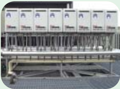
Water heater manifold installation (Australia)
