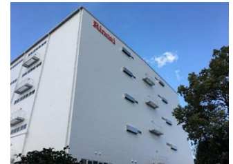
East Japan Logistics Center (Atsugi City, Kanagawa Prefecture)
