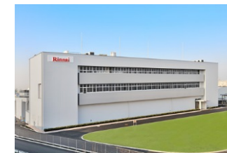
Production Technology Center
