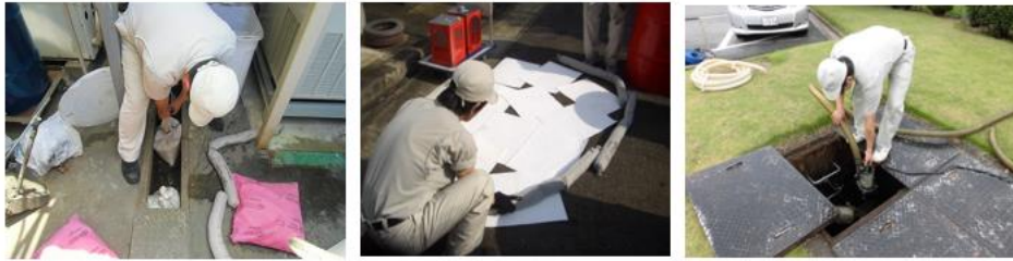
Emergency response drill
