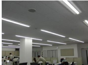
LED lights installed
