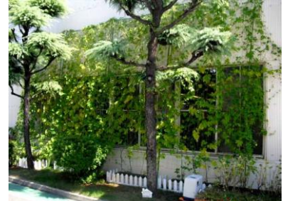
A green “curtain” of plants at one of our offices
