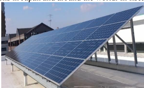
Photovoltaic system (Tohoku sales branch)
