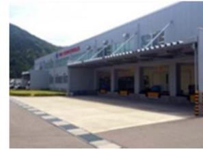
RB Controls, logistics center
