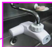
(3) Saved water by installing sensors
