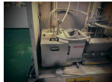
Paint capture equipment installed
