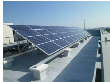
Photovoltaic system (Technology Center)
