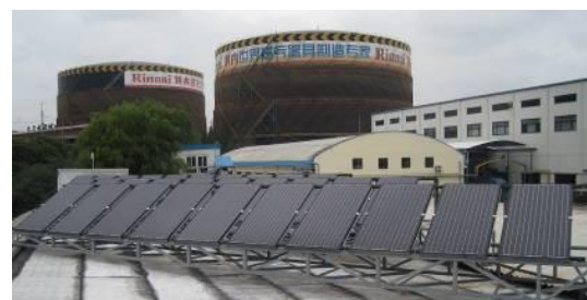
Photovoltaic system and solar waterheating (Shanghai Rinnai Co., Ltd.)
