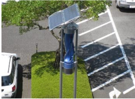
Wind and photovoltaic system (head office parking area)
