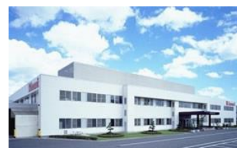
Head office and Komaki Factory
