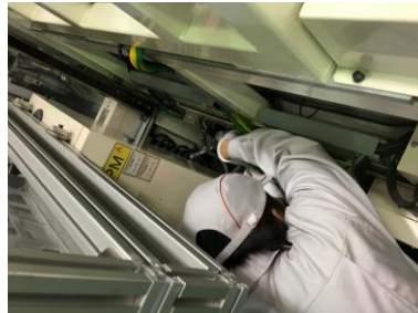
A patrol checking for air leaks (RT Engineering)
