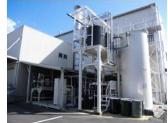
Wastewater treatment plant (Yanagisawa Factory)
