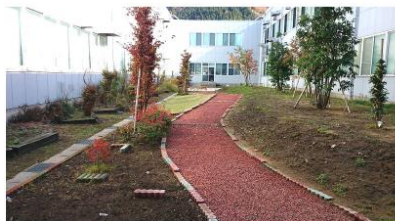
Pathway of crushed roof tiles
