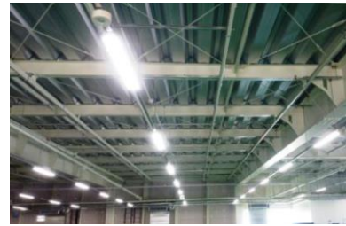
LED lights installed
