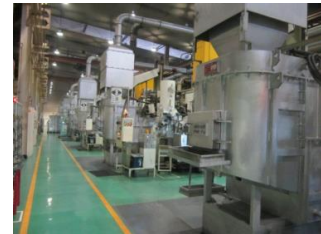
Cast melting furnaces
