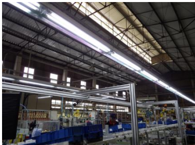
Replacement of conventional lights with LED ones (Rinnai Brazil)
