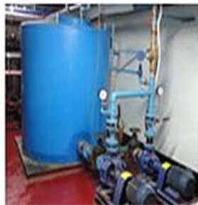
Filtration/storage (tank and transfer pump)
