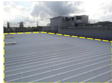
Area of the roof coated (corrugated panels on Factory 1)
