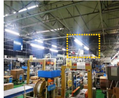
Upgraded fluorescent lights
