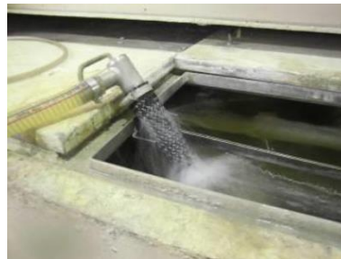
Pre-coating treatment (filtration system)
