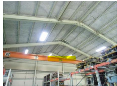
Warehouse (High efficiency lamps)
