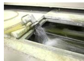
Pre-coating treatment (filtration system)
