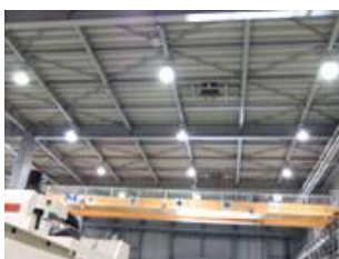
Upgrading to high-efficiency lamps (Production and Technology Development Center)
