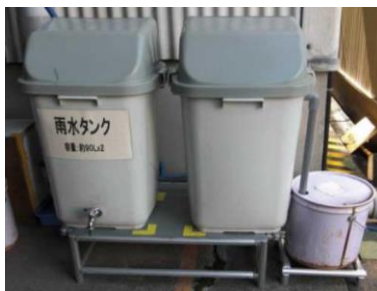
Rainwater tanks
