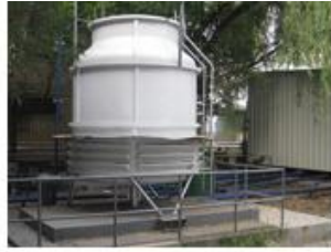
Chiller (cooling tower)
