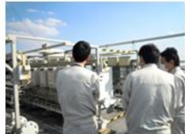
Trainees receive explanations on our water recycling system
