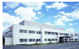
Head office and Komaki Factory
