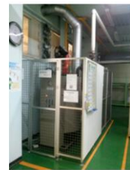
Industrial boiler for the rinse water
