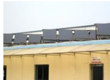
Solar water-heating system
