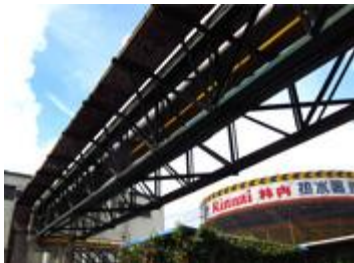
Steam pipes running between facilities
