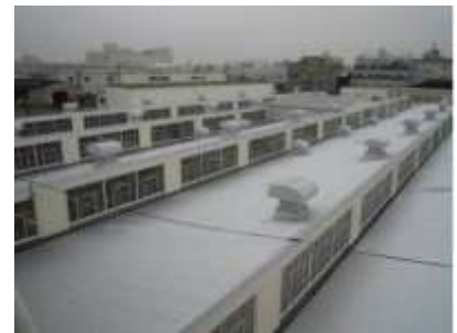
Boards with a heat shield coating installed on the roof
