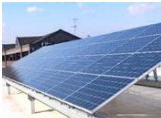
Installing a solar power generation system (Tohoku Branch) Power generated: 6,902 kWh Reduction in CO 2 emissions: Approx. 3 tons (Sept-Mar)
