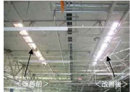
[Before] [After] Sufficient light coming into factory
