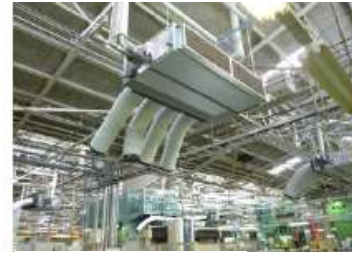
Air conditioning outlets
