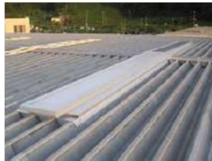
[After] Multilayer polycarbonate skylights to let more light in
