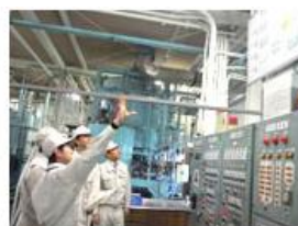
Explanation of wastewater treatment facilities
