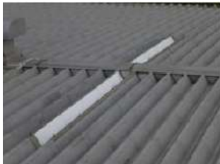
[Before] Previous skylights
