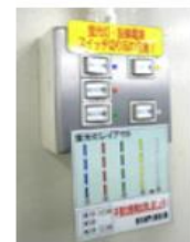
Clearly labelling switches for fluorescent lights (Rinnai Precision)
