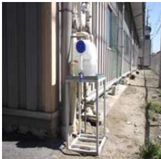
Equipped with a rainwater tank
