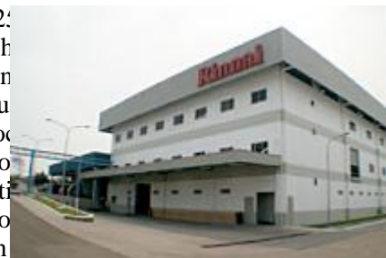
PT. Rinnai Indonesia’s Cikupa Plant
