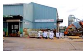
Plant where recycling demonstration tests are conducted
