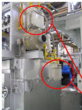
Gas meters are mounted separately.
