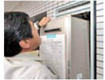
Installing a hot-water unit
