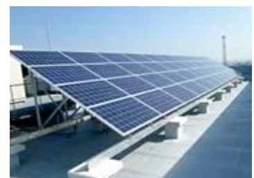
Solar generator panels
