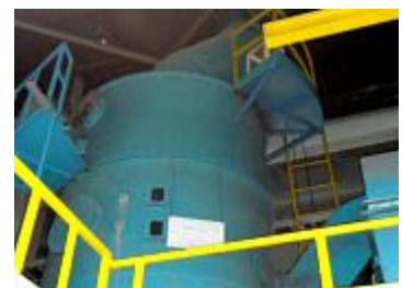
Waste water treatment facilities of Rinnai Korea Corporation
