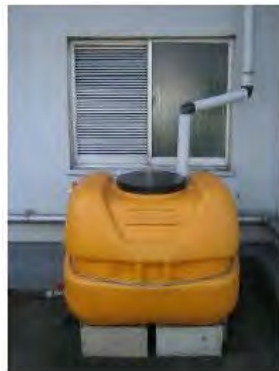
This tank is used to store rainwater.
