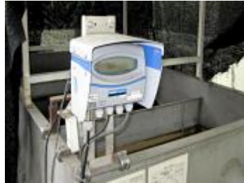
Water quality monitoring equipment
