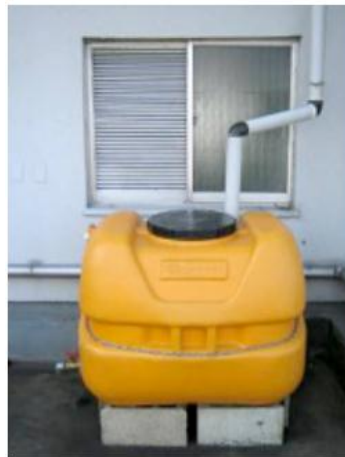
Stored rainwater is used for the vegetable garden on the roof (Aichi Factory)
