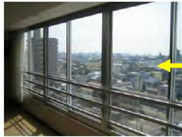
The windows with the heat-barrier film on it
