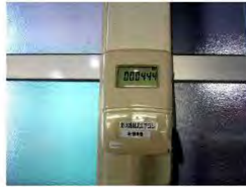
Water meter receiver
