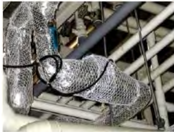
Remote water meter transmitter
