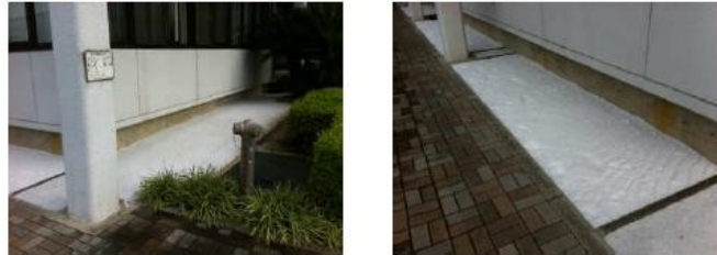
Landscaping materials using calcium carbonate in powder form (*The photographs were taken at Rinnai Corporation's Technology Development Center)
