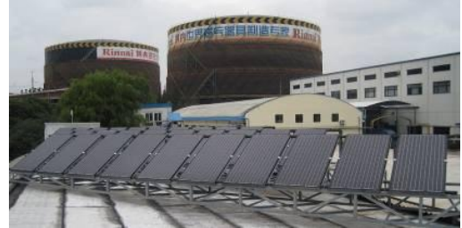
Solar heat panel and photovoltaic panels
