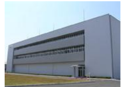
Production Technology Center
