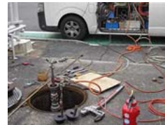
Leak inspection of underground tank (Yanagisawa Manufacturing Co., Ltd.)
