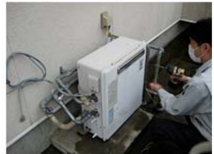
Repair at the affected area
