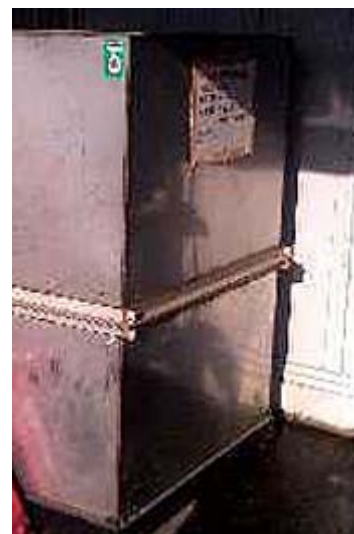
Oguchi Factory Storage for electric appliances in which a trace of PCB was found
